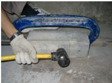
Figure 3: Hacking with air tool hammer
