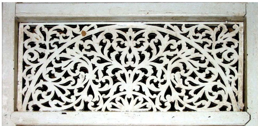
Figure 1.0: Ventilation panel on top of a window of Tengku Long's house in Kuala Terengganu
