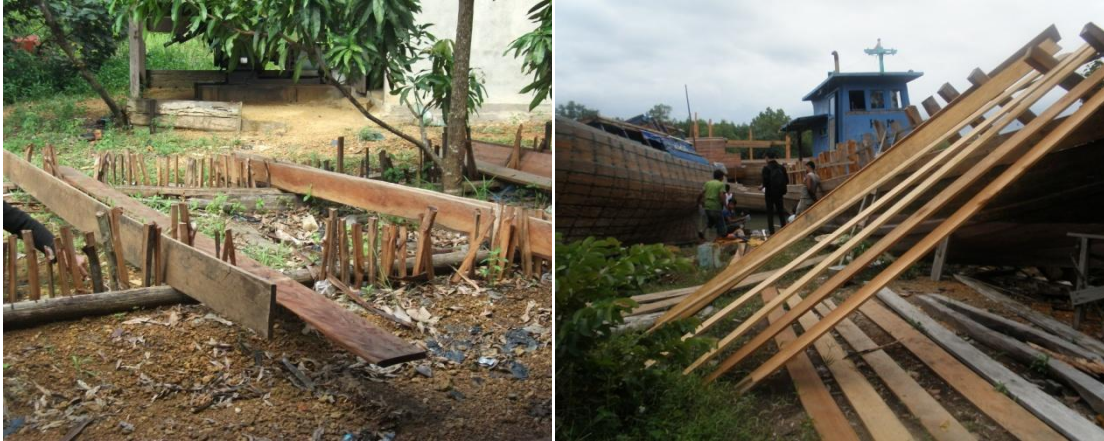
Figure1.1: Drying lumber issue in traditional ship production in Kepulauan Riau, Indonesia.
