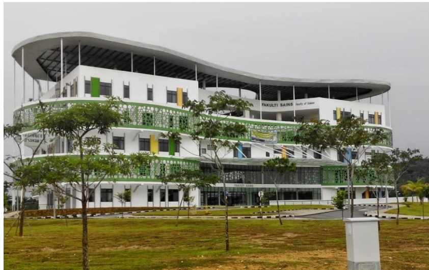
Figure 1.1 T05 UTM Space building
