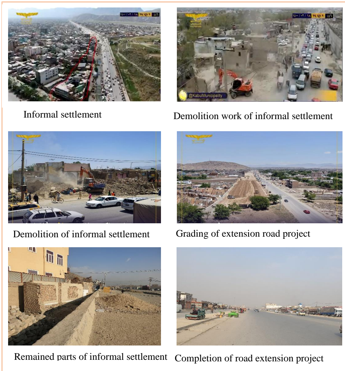
Figure 1.2 Demolition of informal settlement and new constructed roads.
