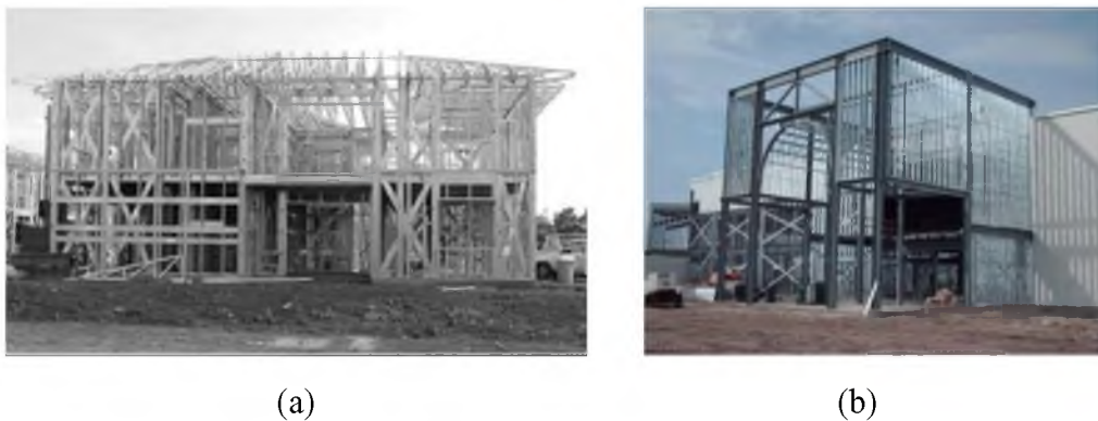
Figure 1.2 (a) A CFS wall system (Alliance, 2007) and (b) a multi-story building structure used CFS as the wall system's main structure from steel profiles ( www.greenmaltese.com ).
