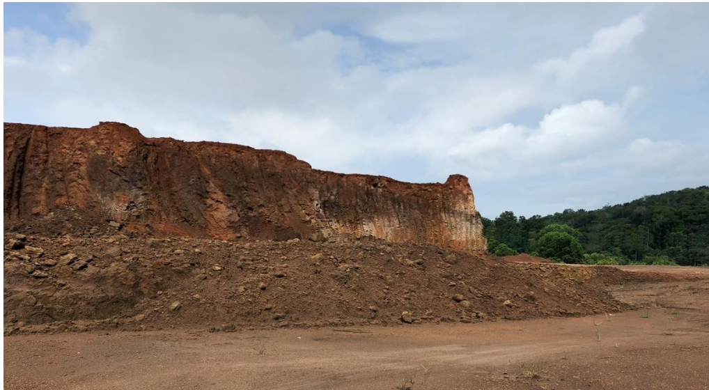
Figure 3. Ground condition at Semambu.
