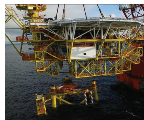
Figure 8. Offshore topside installation in oil and gas development phase
