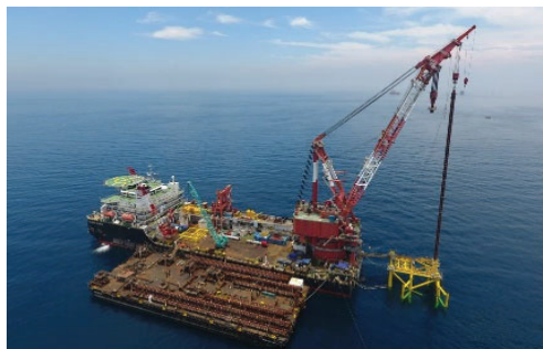
Figure 6. Offshore platform jacket installation in oil and gas field development phase
