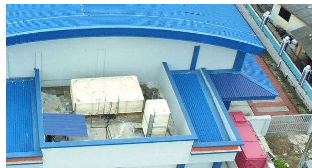
Figure 10. Inaccessible area for TLS which UAV can cover
