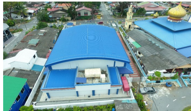
Figure 9. Rooftop area covered by UAV
