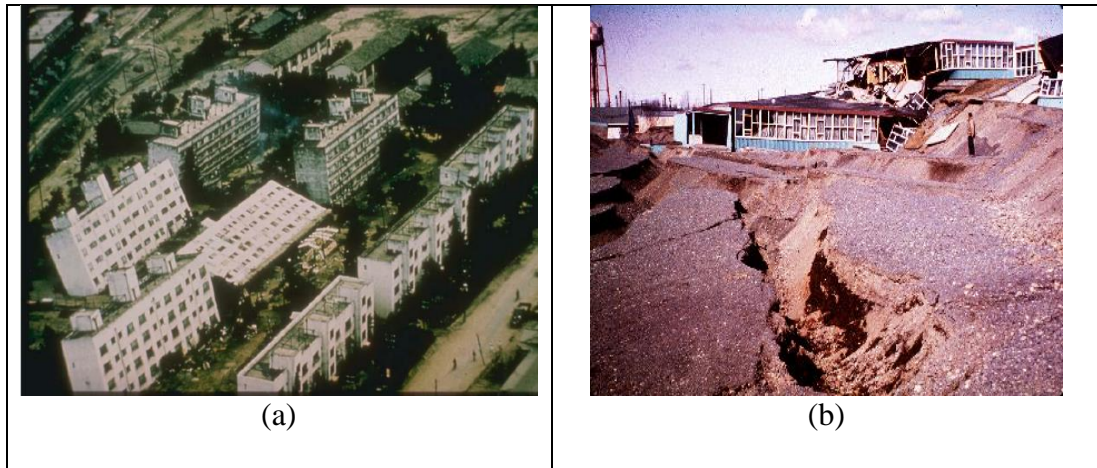
Figure 1.1 Digital images showing damages caused by soil liquefaction (a) Failure of apartment buildings by tilting in Niigata due to liquefaction (b) Failure of roads leading to a Government Hill elementary school in Alaska due to liquefaction (Source: National Geophysical Data centre cited by Agaiby and Ahmed (2016))
