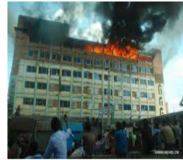
Figure 3: Exterior and interior of after fire broke out at factory buildings at Gazipur. (Source: The new work times)
