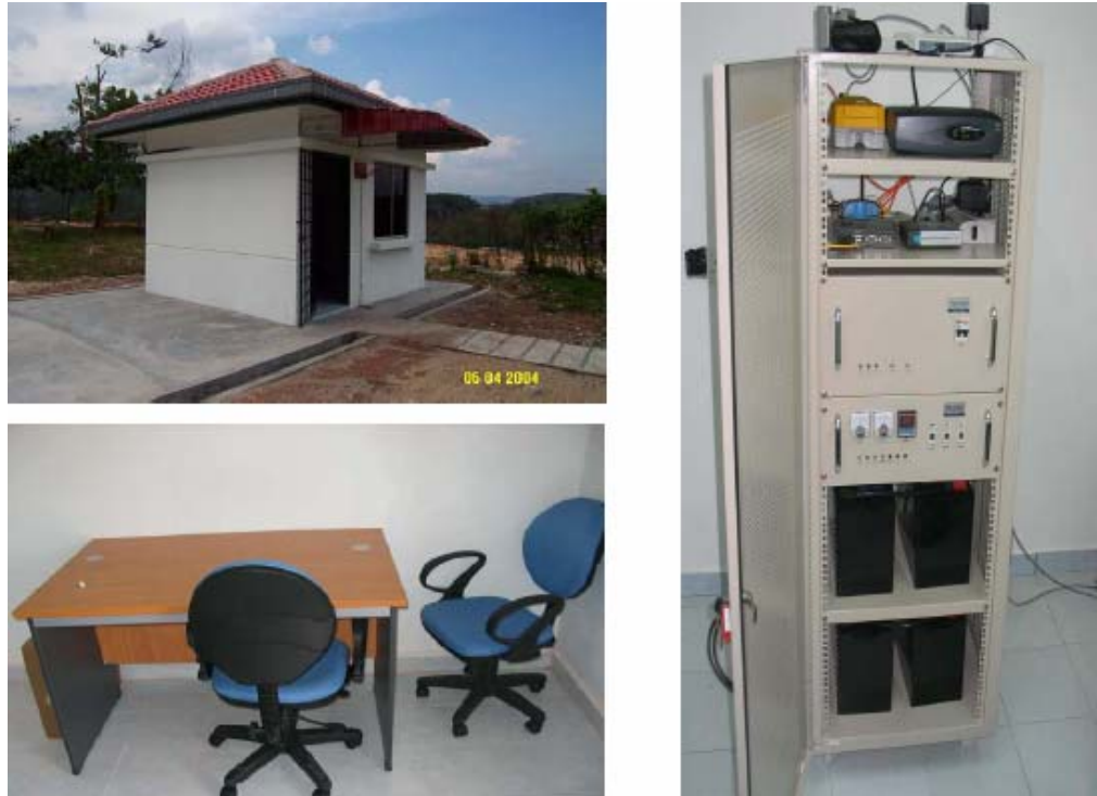
Figure 3.16: Example of Reference Station Cabin and Equipment
