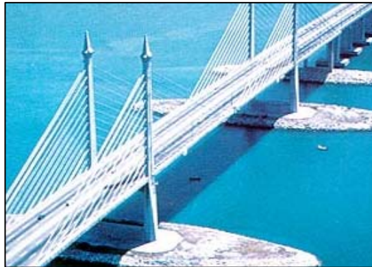
Figure 2.15: Penang Bridge, Penang
