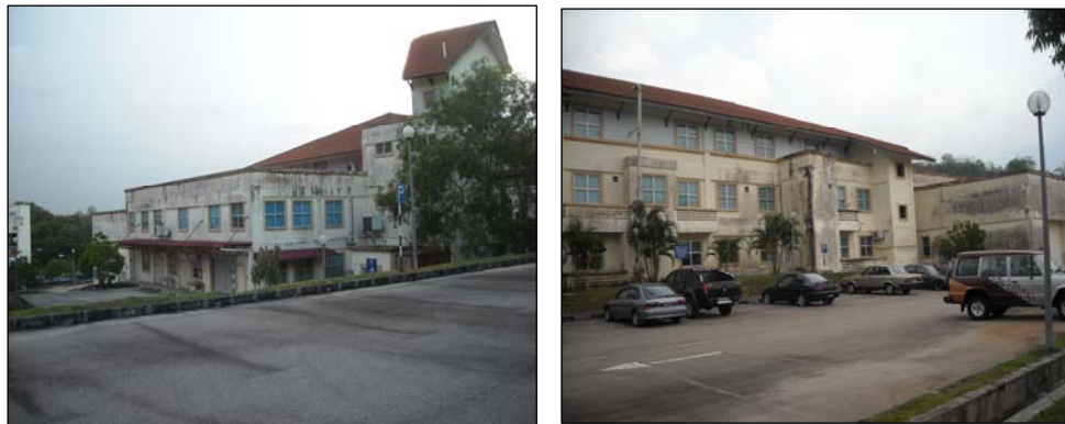
Figure 5.12: Overview of P23 Building
