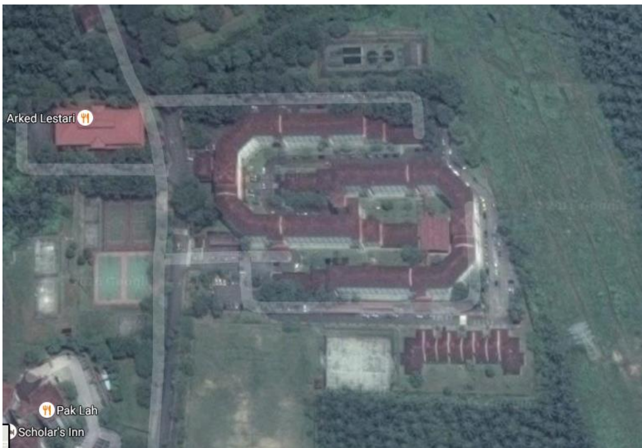
Figure 1. Kolej 9, UTM, Skudai (The test bed)
