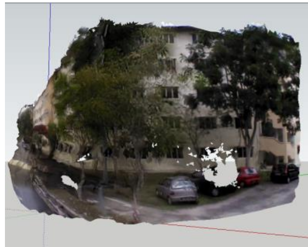
Figure 4. Low quality 3D model along with all the obstacles such as trees and vehicles after editing via SketchUp Trimble.
