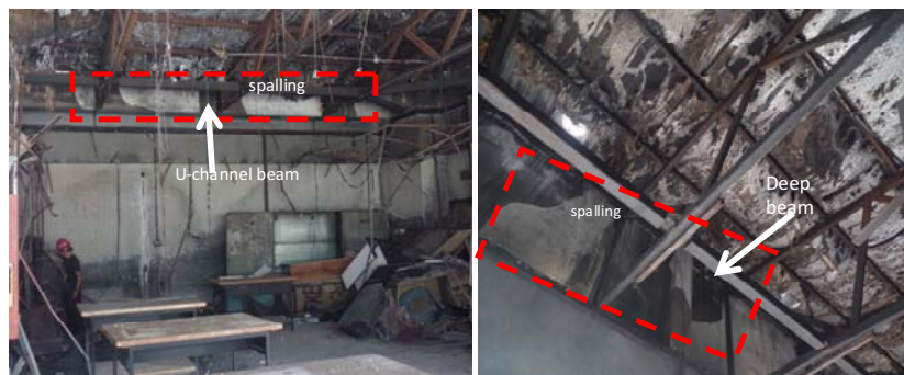
Figure 6. Physical appearance of the beams
