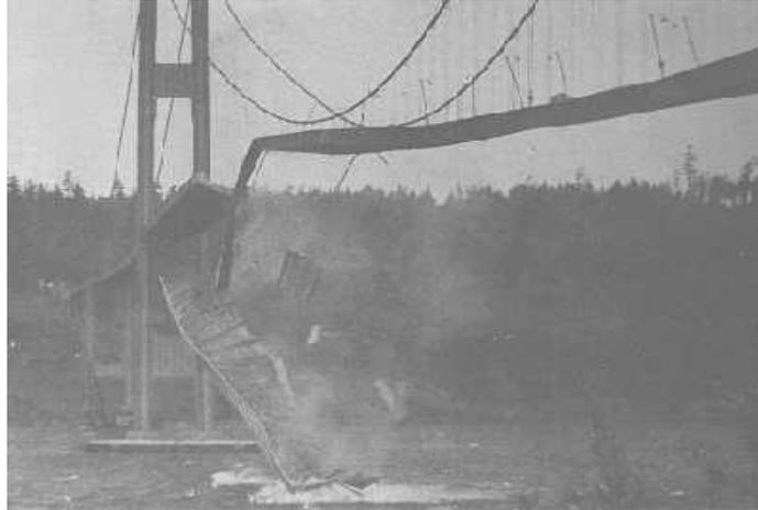
Figure 4.7: Failure of the Tacoma Bridge
