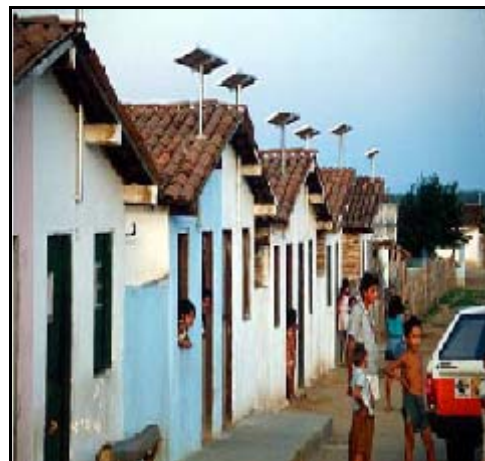
Figure 1.3: Stand-alone rural electrification
