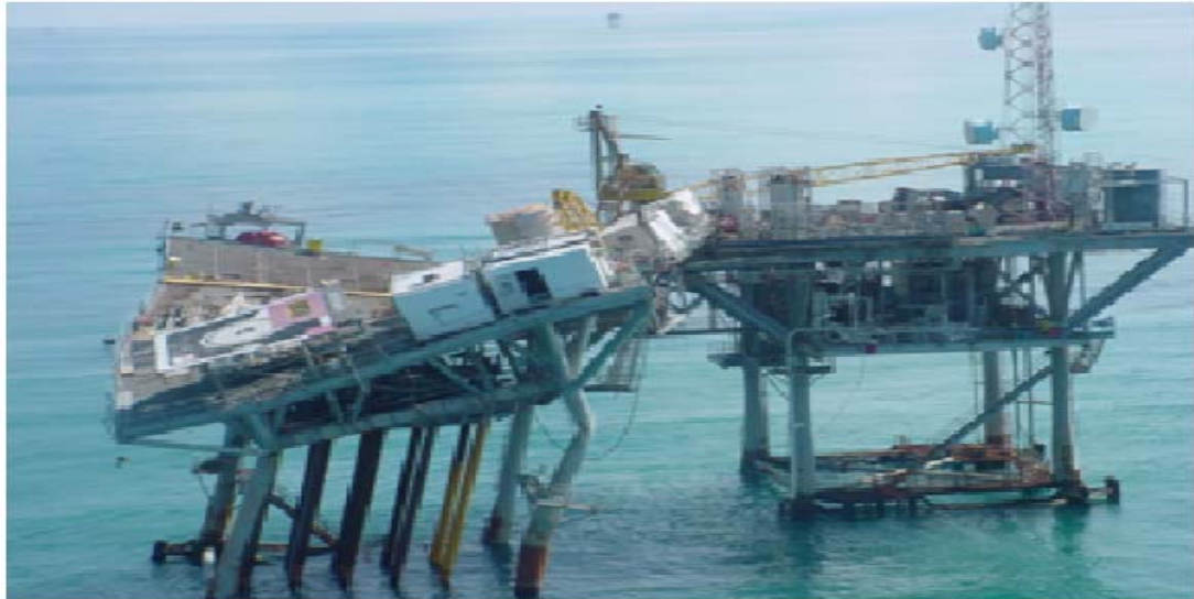
Figure 1.3: Hurricane Lily's impact on fixed platform
