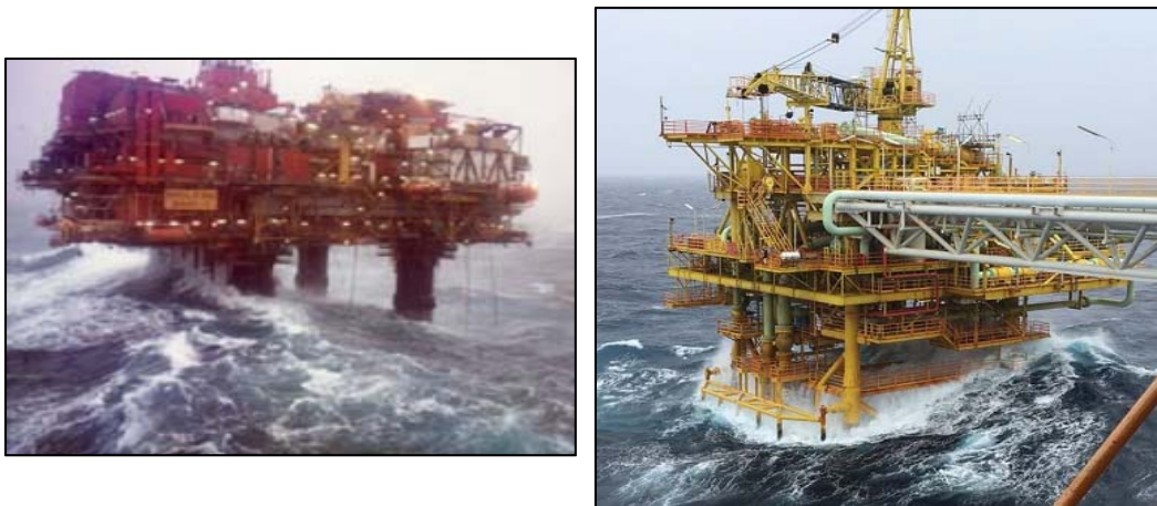
Figure 1.6: Actual photos of wave-in-deck loading scenario Shell Group of Companies. (2013)
