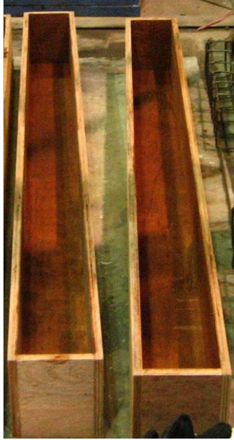
Figure 3.21: Wooden formwork for reinforced concrete beam.
