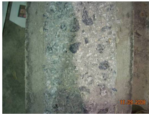
Figure 3.24: The bottom surface of the concrete beam is roughened to provide better bonding.
