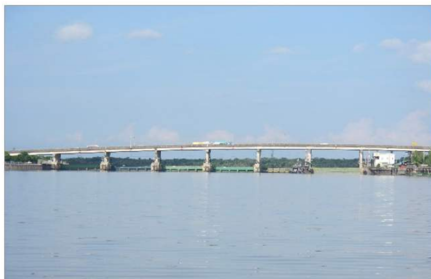
Figure 22. The tidal barrier to prevent seawater intrusion impact, Sarawak [142]. Reprinted from Saline Water Intrusion through Rajang River Network due to Sea Level Rise, 2019; open access publication by IOSR Journals.
