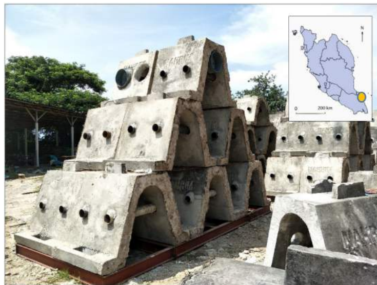
Figure 12. WABCORE as a wave breaker and artificial reef structure
