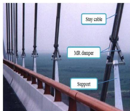
Figure 2: MR damper on cable bridge [5]
