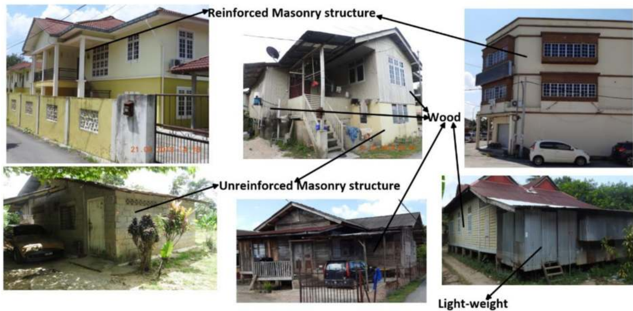
Figure 12. Examples of different building construction type and materials in Kota Bharu, Kelantan.
