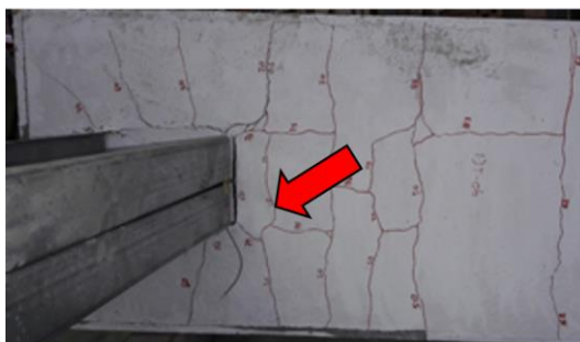
(c) IJT-06 first crack
