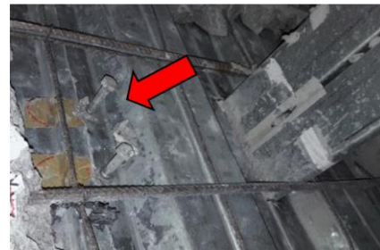
(b) IJT-03 shear connector
