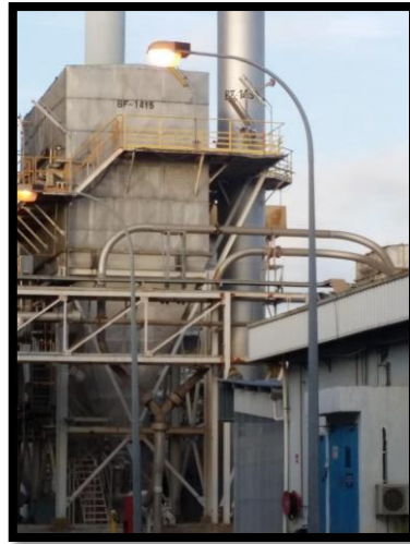
Figure 1.2 Street lighting condition
