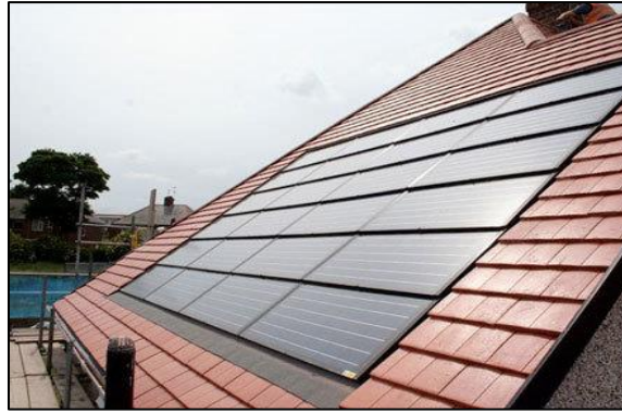
Figure 1.4 Rectangular Shape PV Panels Integrated with Conventional Roof
