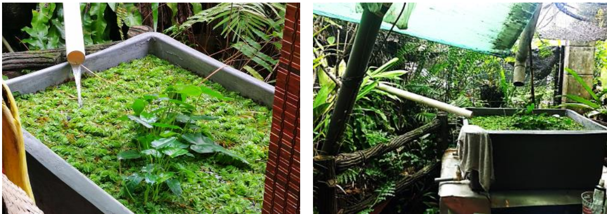
Figure 9. The rain water harvesting system with bio-organic treatment
