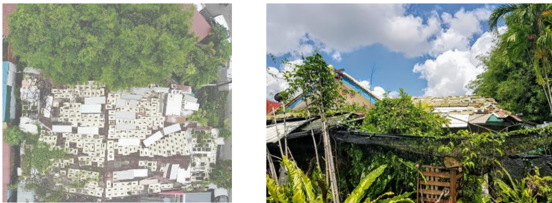
Figure 6. The polystyrene or polyfoam covers insulating the roof and creating the green roof
