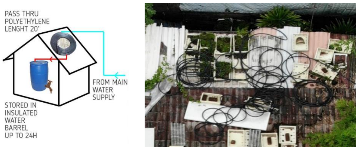
Figure 7. Thermal hot water system using coil of black pipes placed on the roof
