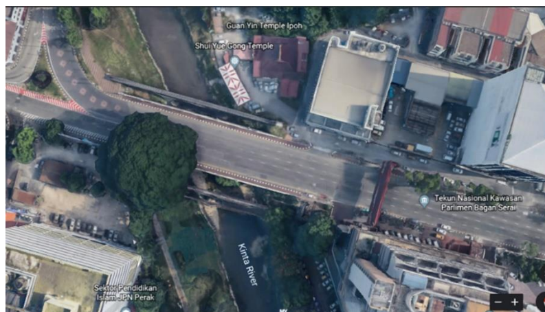
Figure 4. Sultan Idris Shah Bridge in Ipoh, Perak, Malaysia
