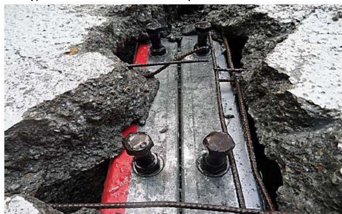
Figure 7. M16 bolted shear connector condition after test.
