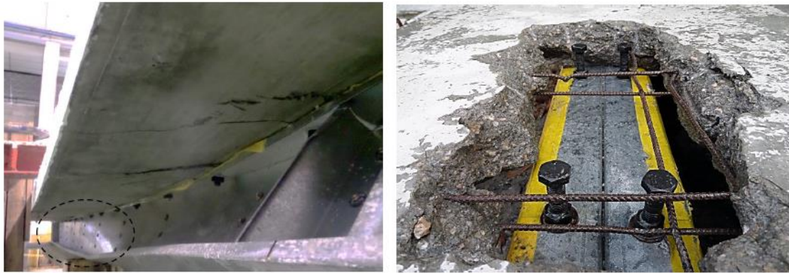
(c) CFS web buckling
