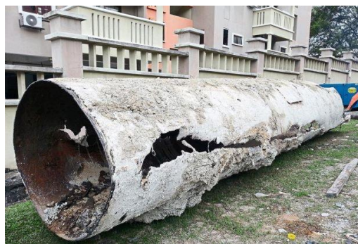
Figure 1. Old sewerage after the excavation in Puchong. (Source: The Star newspaper)
