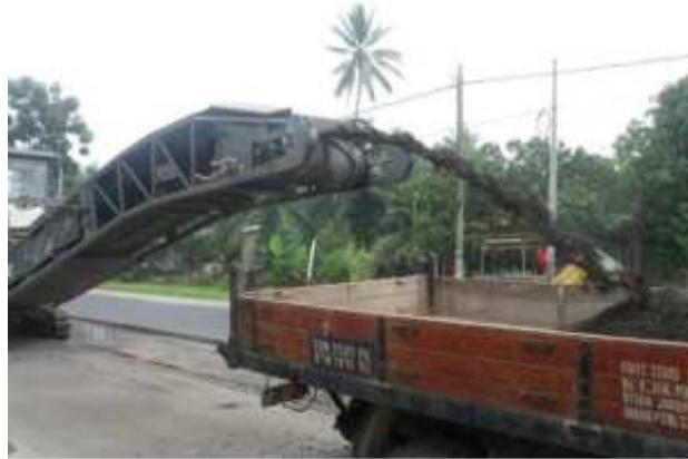
Figure 2. Cold milling process
