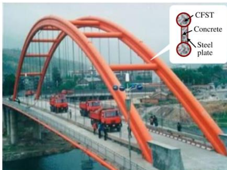
Figure 1.6 Wangcang East river bridge China
