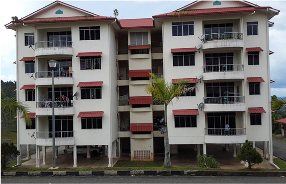
Figure 1.4 RC building with "pilotis" configuration in the affected area. (Alih & Vafaei, 2019)
