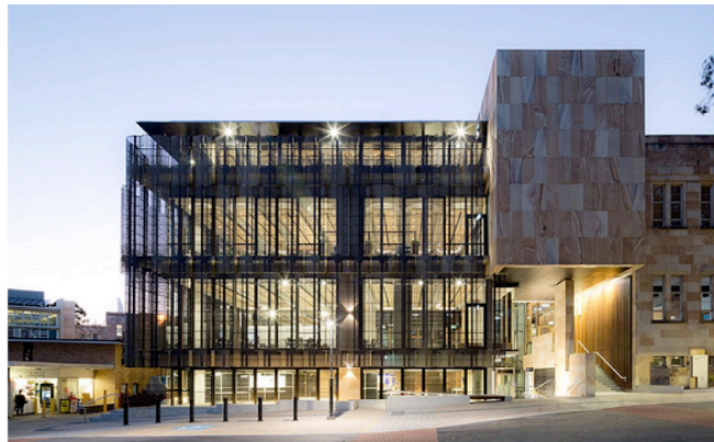
Figure 1. Structural geopolymer concrete in Queensland's University (Global Change Institute) with three suspended floors [4].
