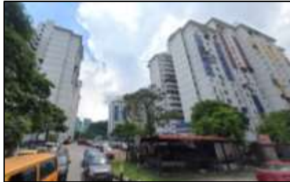
Photo 3: PPR Kerinchi Lembah Pantai residential building
