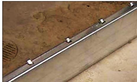
(b) Bent-up tabs on CFS flange
