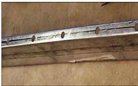
(a) Pre-drilled holes on CFS flange
