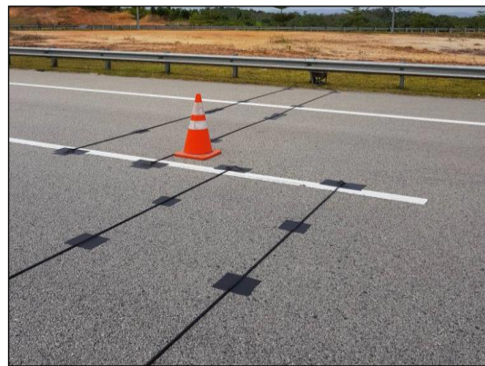
Figure 2. Pneumatic tubes laid across the traffic lanes.
