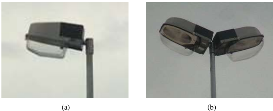
Figure 1: Photo of (a) 250W and (b) 400W street lighting lantern
