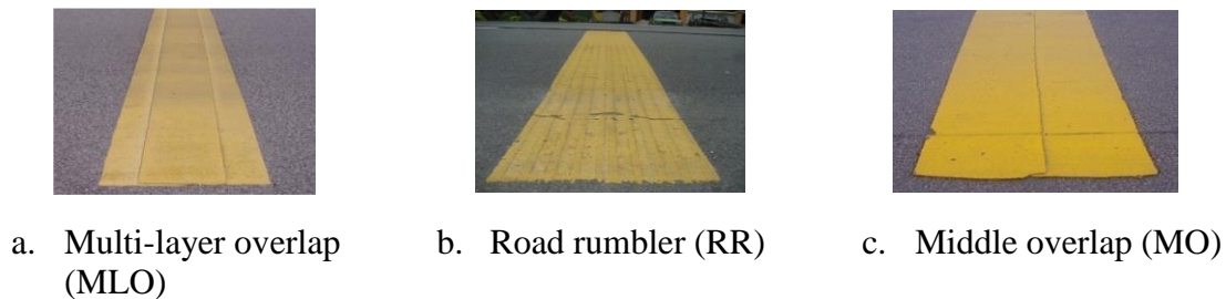
Figure 1. Types of thermoplastic rumble strips profiles.
