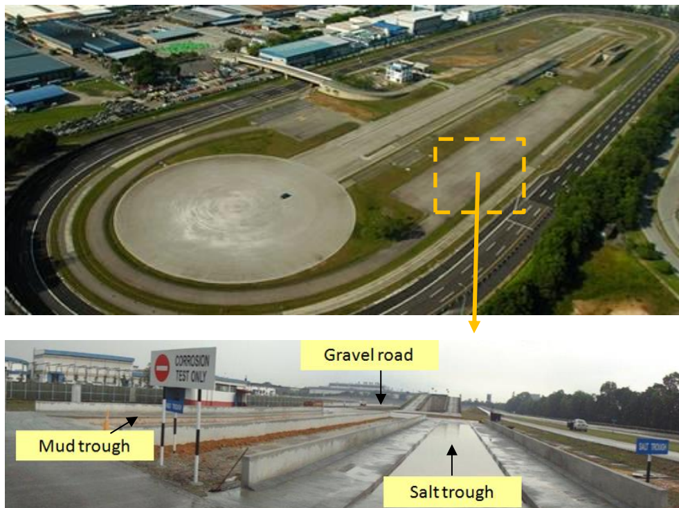
Figure 2. PROTON Test Track and Corrosion test facilities.
