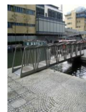
(c) Pedestrian bridge
