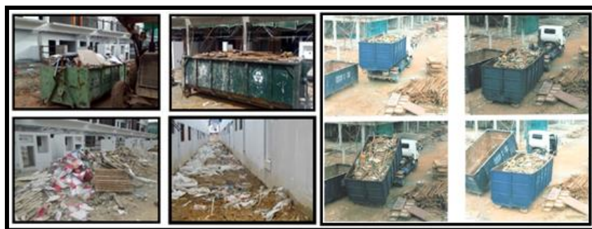
Figure 1. Construction waste disposal process (adapted from EMS 14001 records).
