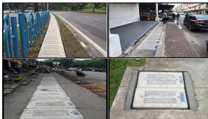
Figure 7. Implementation of eco-composite porous concrete drainage covers in Shah Alam, Selangor.
