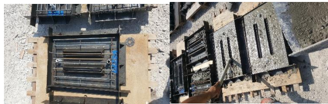
Figure 5. Preparation of porous concrete for drainage cover.
