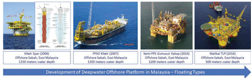
Figure 1. Development of deep-water offshore platform in Malaysia—floating types.
