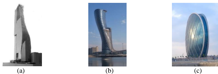
Figure 3. (a) Phare Tower in Paris (b) the Capital Gate in Dubai and (c) Aldar Headquarters in Dubai.
