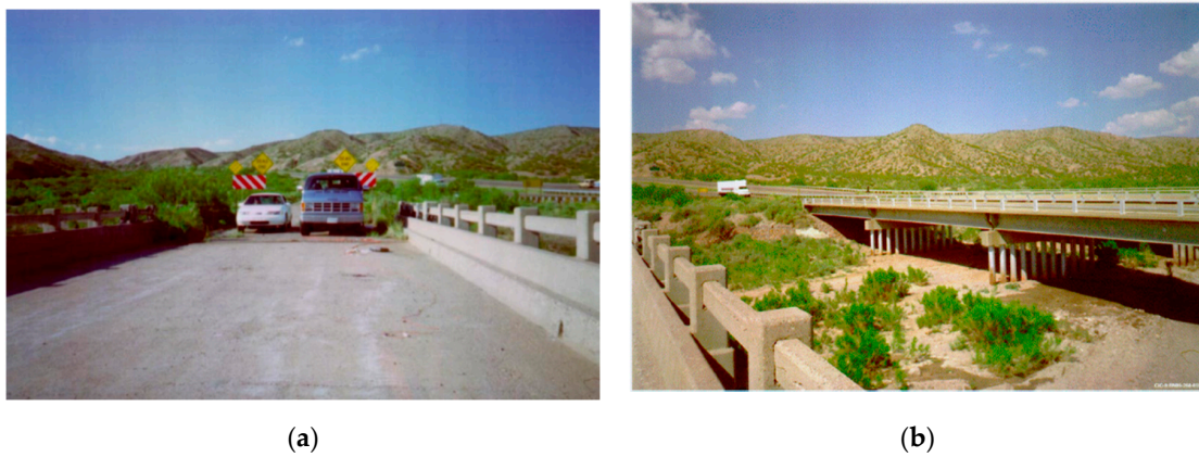
Figure 9. The ambient testing of the Alamosa Canyon Bridge. (a) Crossing of vehicles over the bridge. (b) Passing vehicle from the adjacent bridge [46].
