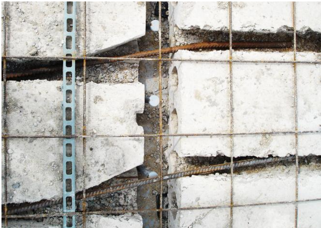
Figure 1.2 Bending of the coupling bars
