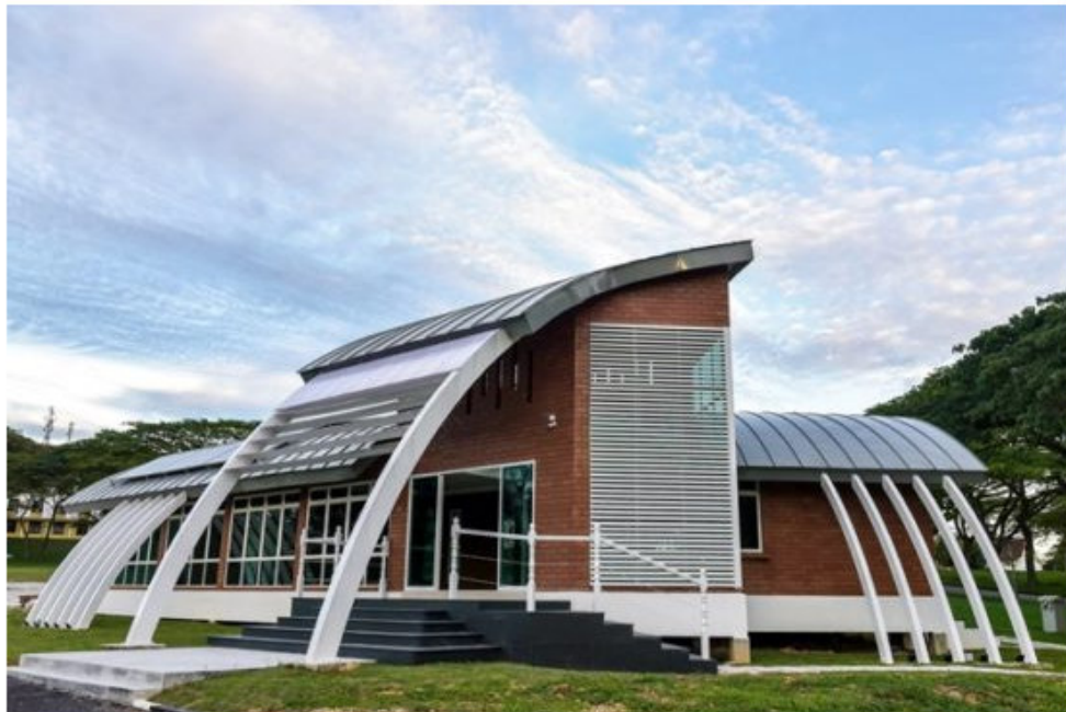
Figure 1.1 : The UTM Eco-Home building.
