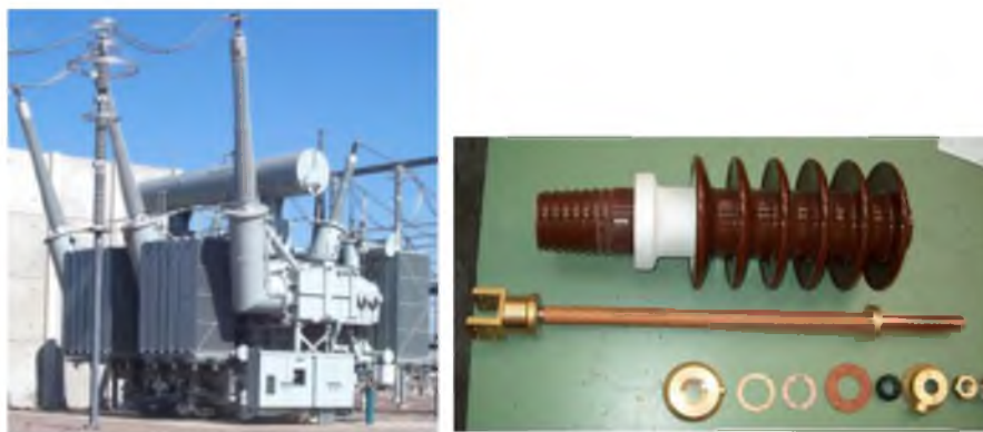
Figure 1.2 Power transformer HV and LV bushing
