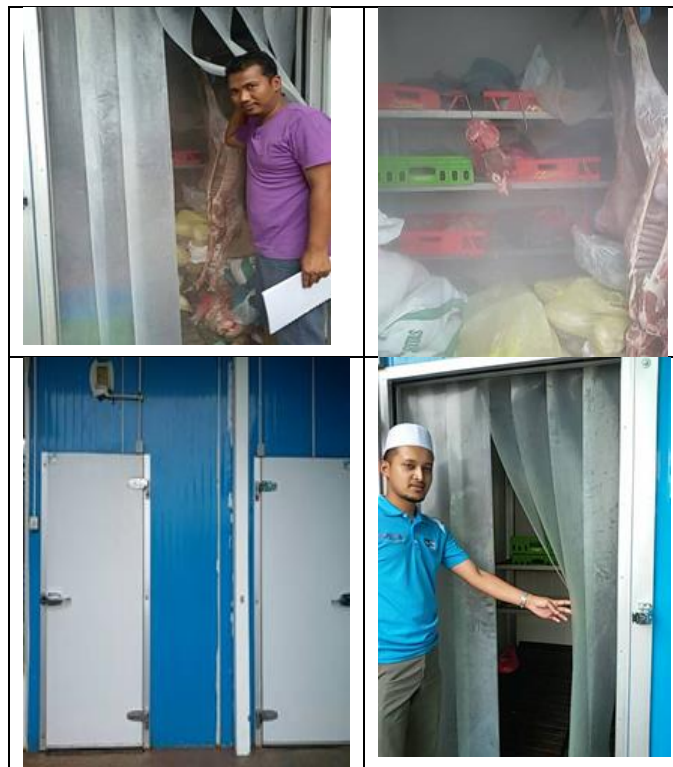
Images 4.4: Freezer, Chiller, and Refrigerator
