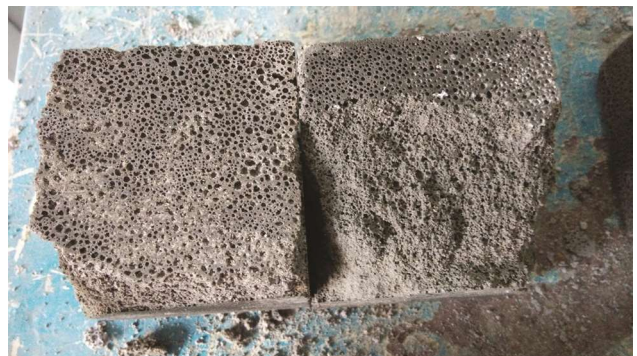
Fig. 3 — Voids formed in hardened LFC
