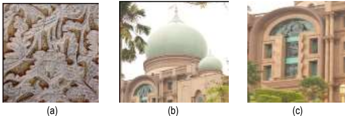
Figure 6: (a) Stone granite (b) Green fiber-glass dome (c) Wrought iron grill and detailing (Source: Author)
